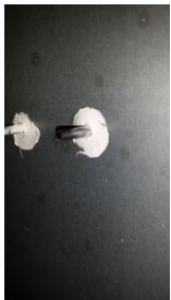
Pressure tap, not in flush with the internal casing
